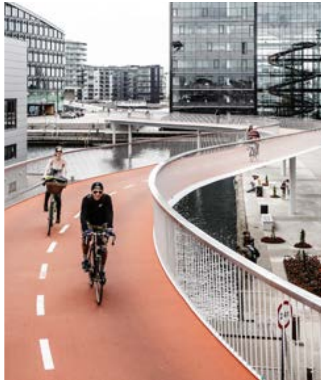
Cykelslangen in Copenhagen Dissing+ Weitling Architecture In cooperation with Rambøll and MT Højgaard Photo: Rasmus Hjørtshøj - COAST Studios
